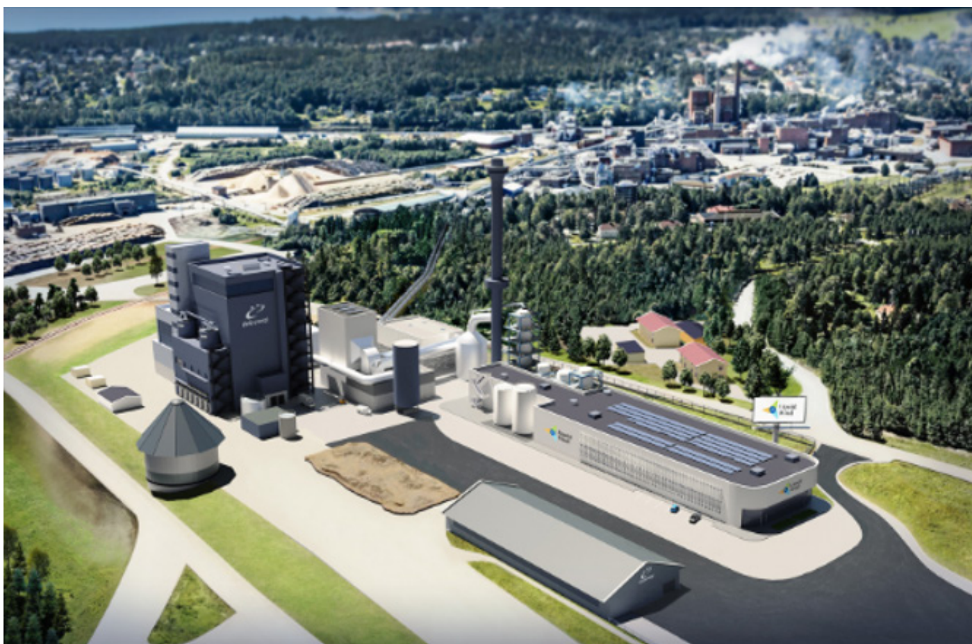
Integrated solutions examples from Top to bottom: Palopuro Agroecological Symbiosis in Finland 39 , Bakkafrost Førka refinery in the Faroe Islands 40 , Liquid Wind FlagshipONE in Sweden 41 .
